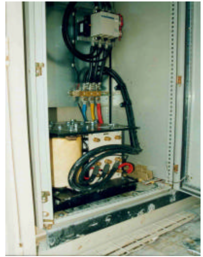
TYPICAL INSTALLATION IN A 300kW STARTER
